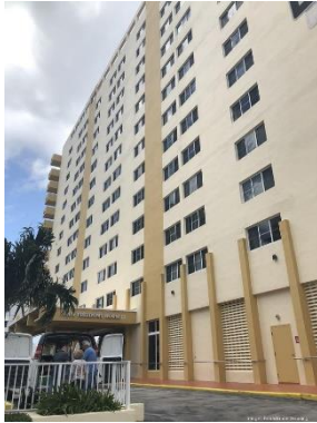
Foundation Housing acquired Four Freedoms House in Miami Beach
